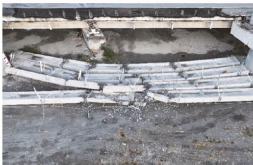
(c) P1 ~ P2 間預力大梁掉落
