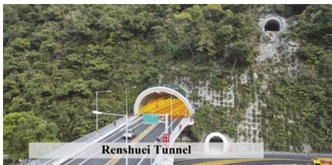
Main Tunnel, Excavation Tunnel, and Smoke Extraction Tunnel for the Renshuei Tunnel with Two-way Traffic in a Single Tube
