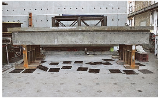
(a) 鋼板放樣鑽孔
