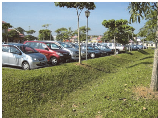
(e) Ecological swale after completion
