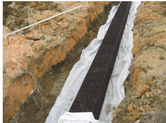
(b) Module is laid in the trench and wrapped in geotextile
