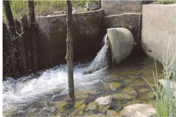
Fig. 10 Check valve used to provide flow in one direction only through a culvert
