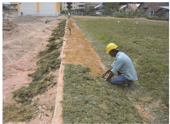
(d) A swale is shaped and topped up with top soil before being turfed
