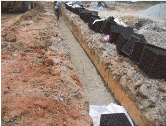
(a) A trench is dug with backhoe and layered with river sand
