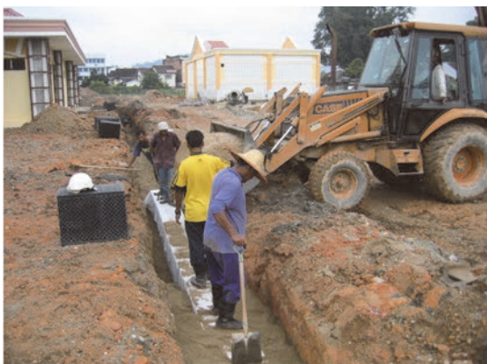
(c) Trench is backfilled with enclosed module buried within
