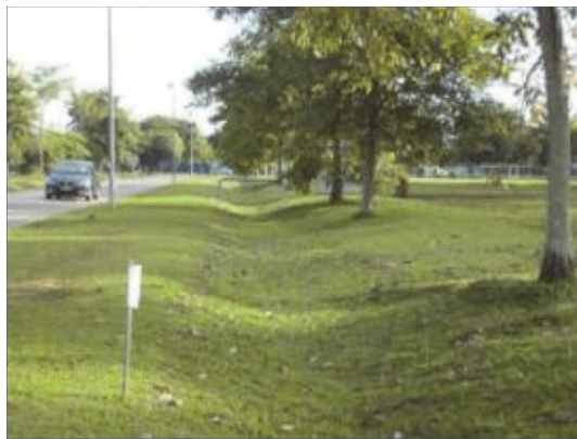
(e) Ecological swale after completion
