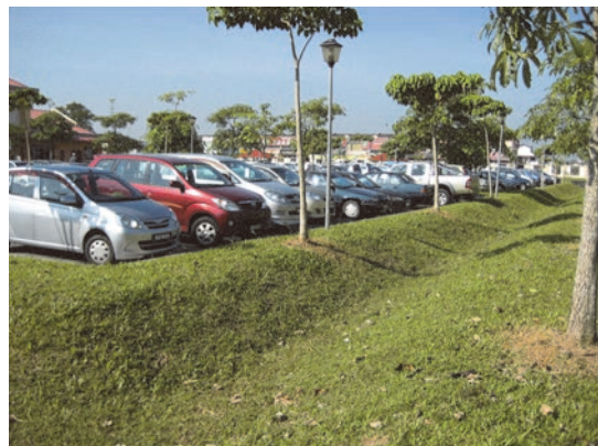
(e) Ecological swale after completion
