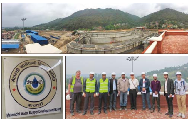
Fig. 4 Site survey Sundarijal water treatment plant project
