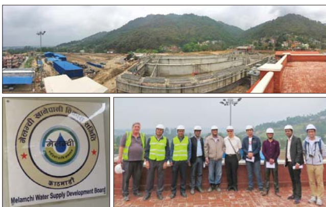
Fig. 4 Site survey Sundarijal water treatment plant project
