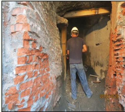
(6) Install internal supplementary braces
