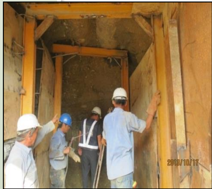
(5) Bracing for excavation
