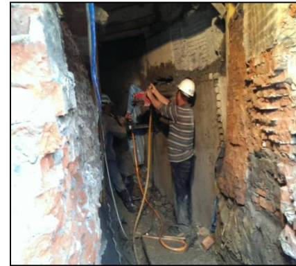
(7) Drill holes to assist in breaking the wall
