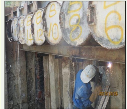
(4) Install supplementary support
