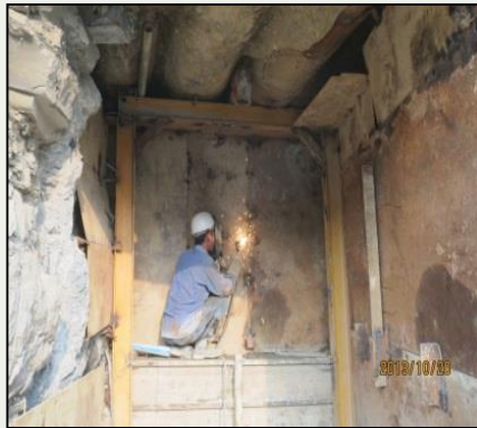
(6) Removal done; seal the contingency tunnel
