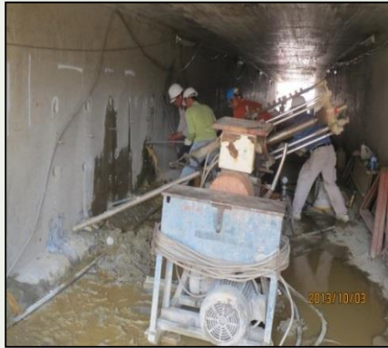
(2) Ground Improvement through the old culvert walls
