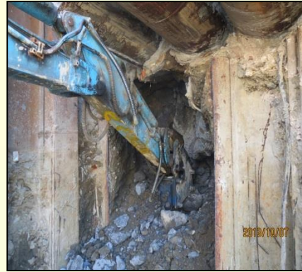
(3) Remove existing wing walls
