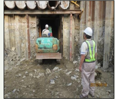
(4) Remove existing wing wall
