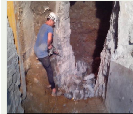
(8) Manually remove existing wing wall
