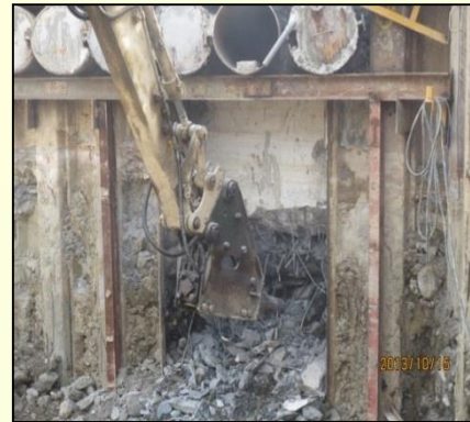
(3) Remove existing retaining wall
