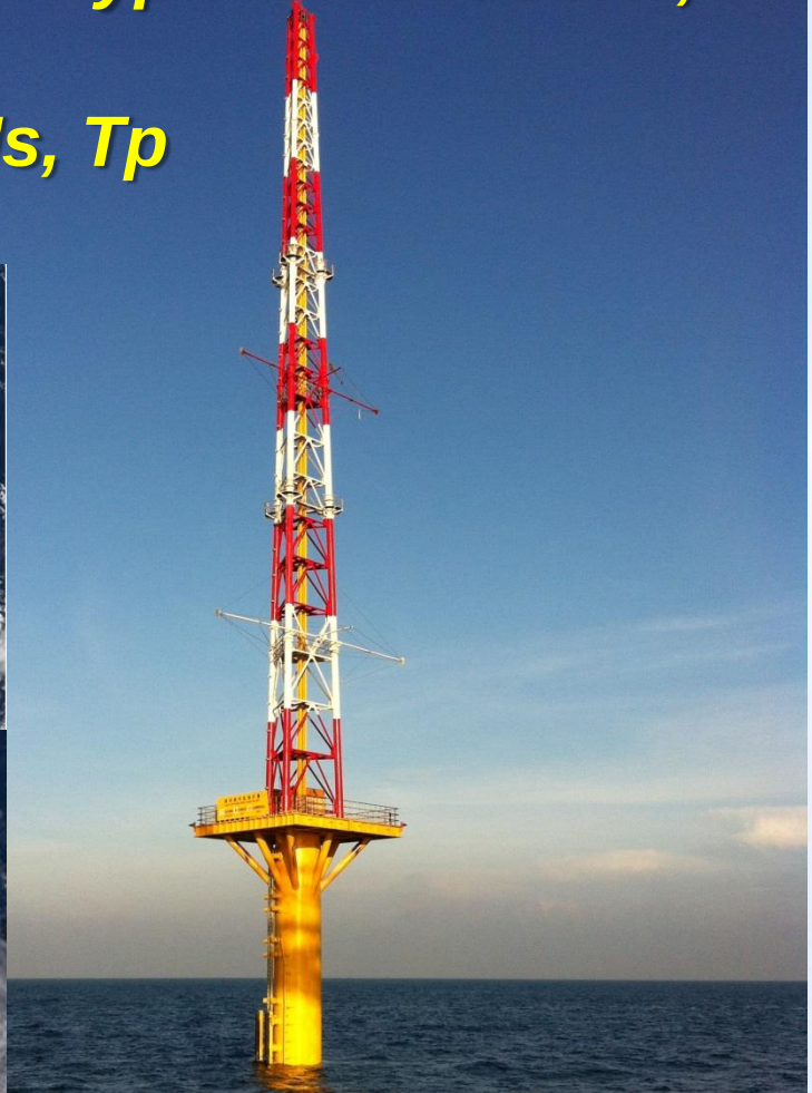
TGC Wind Farm
