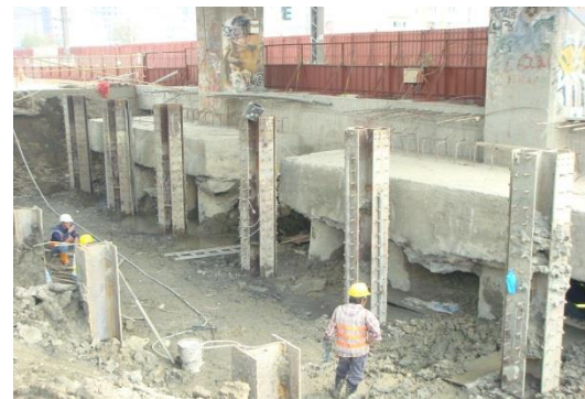
Underpinning Support the Bridge
