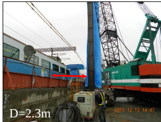
Limited space construction
