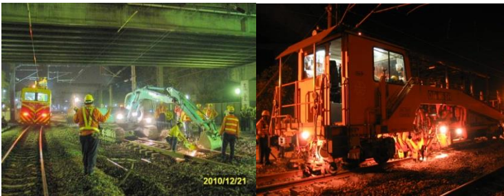
Track & signal shift during 6 Hrs
