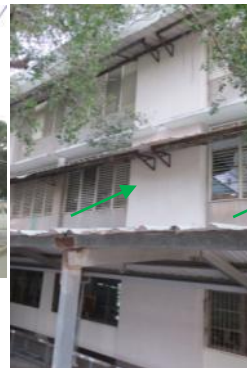
Retrofitted in 2011 ( enlarged columns and wing walls )
