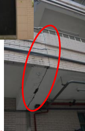
Waiting for seismic retrofit damages along the expansion joint
