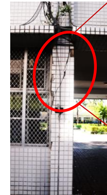
Waiting for seismic retrofit Shear failure of a first-story column
