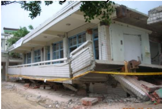
An in-situ test of school building in Taoyuan
