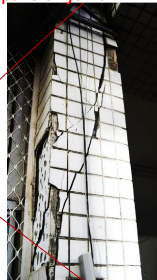
Waiting for seismic retrofit damages along the expansion joint
