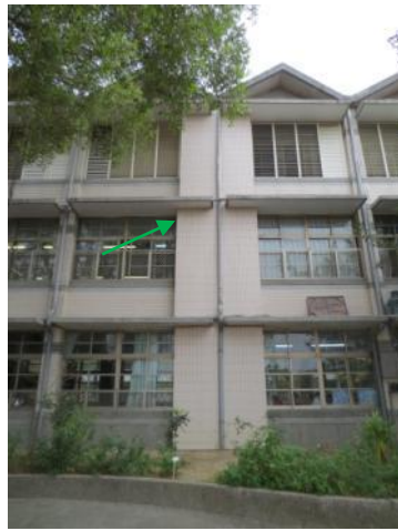
Retrofitted in 2011 ( wing walls )
